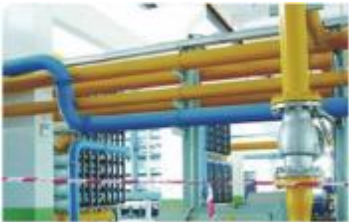
Daishan County Xiushan Seawater Desalination Project
